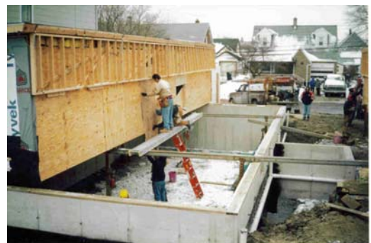
'There's No Place Like Home' construction at 48 Doyle Ave, Buffalo, NY
